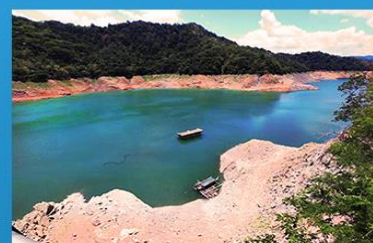
BULACAN BULK WATER SUPPLY PROJECT
