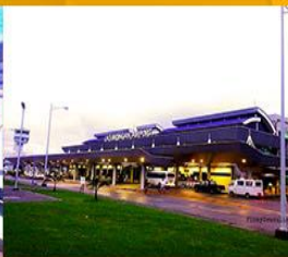
LAGUINDINGAN AIRPORT OPERATIONS, MAINTENANCE & DEVELOPMENT PROJECT
