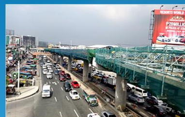
NAIA EXPRESSWAY (PHASE II) PROJECT
