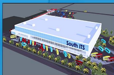
SOUTH INTEGRATED TRANSPORT SYSTEM PROJECT
