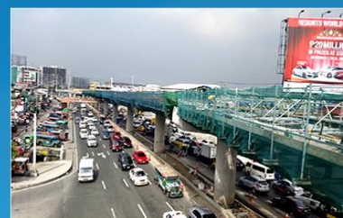
NAIA EXPRESSWAY (PHASE II) PROJECT
