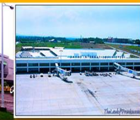
DAVAO AIRPORT OPERATIONS, MAINTENANCE & DEVELOPMENT PROJECT
