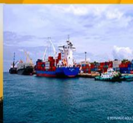
DAVAO SASA PORT MODERNIZATION PROJECT
