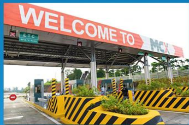
DAANG-HARI-SLEX LINK ROAD PROJECT
