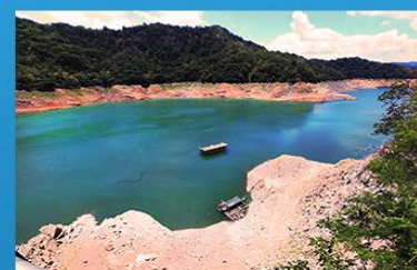
BULACAN BULK WATER SUPPLY PROJECT
